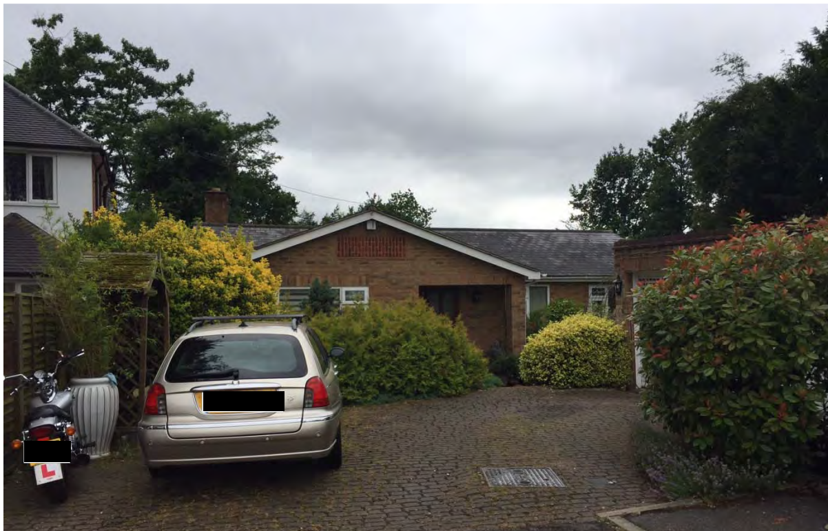
Existing front elevation of the subject property and the neighbouring property No.5a Crest View located to the left.
