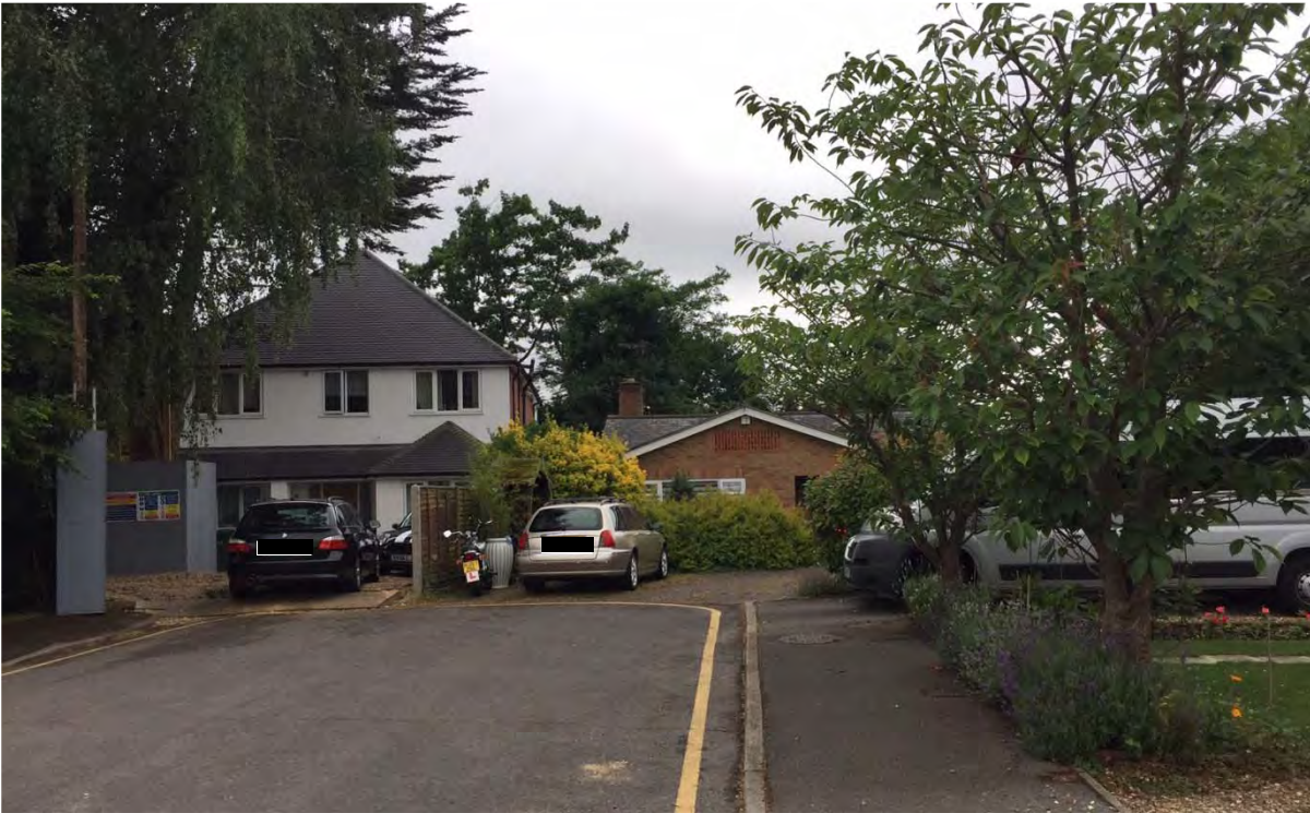
Existing front elevation of the subject property.
